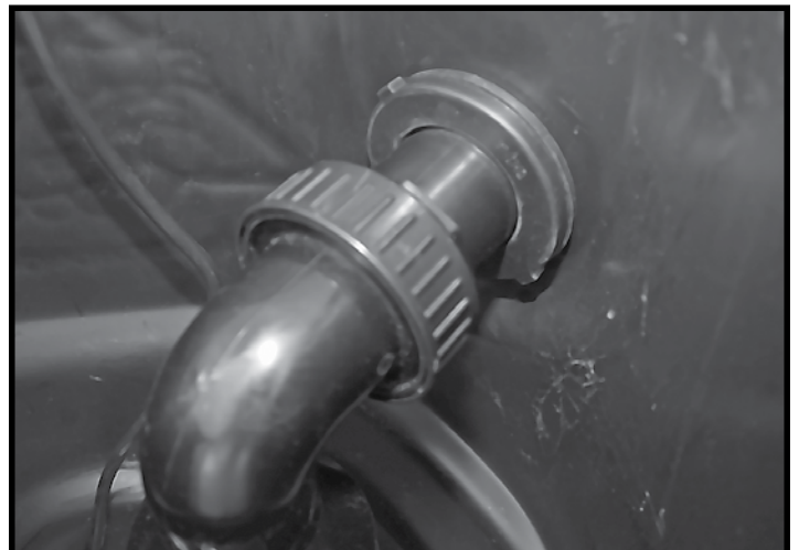
Ex. 15 One adaptor threads directly into the pump, the other threads directly into the bulkhead on the back of the skimmer. Apply silicone or Teflon tape (not included) to the threads of the fitting. NOTE: One pump shown. Your installation may have two pumps.
