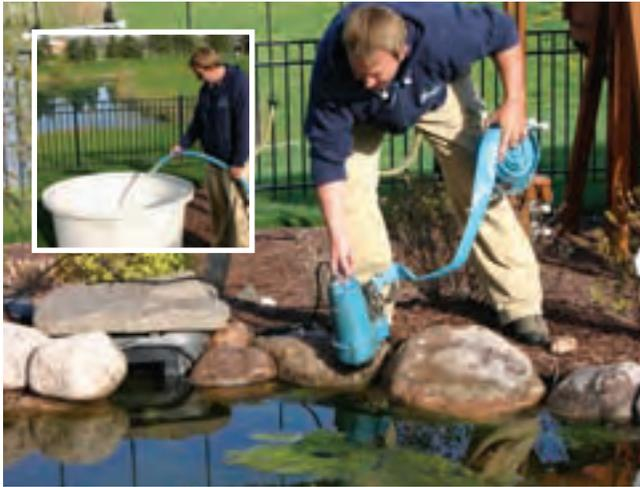
**1** Begin draining the pond with a clean-out pump, or simply use the waterfall pump with chicken wire around it to prevent fish from being sucked into the impeller. Use flexible PVC pipe or a fire hose to discharge the water into the surrounding landscape, relocating the hose two or three times to allow ground seepage. If the
