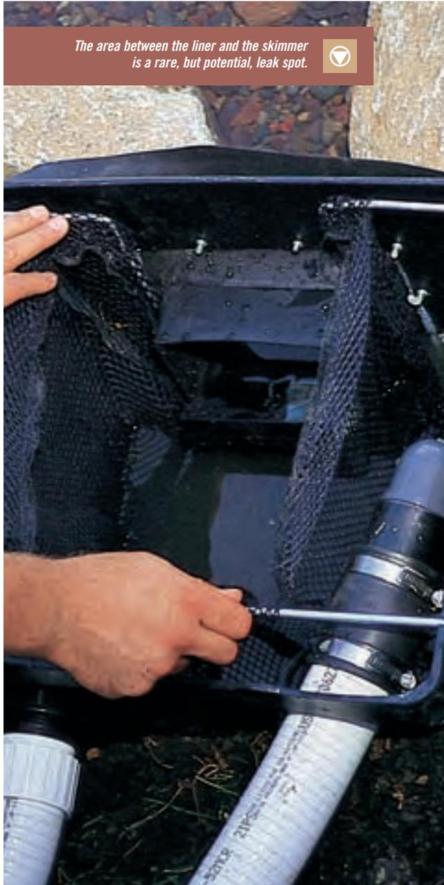
The area between the liner and the skimmer is a rare, but potential, leak spot.
